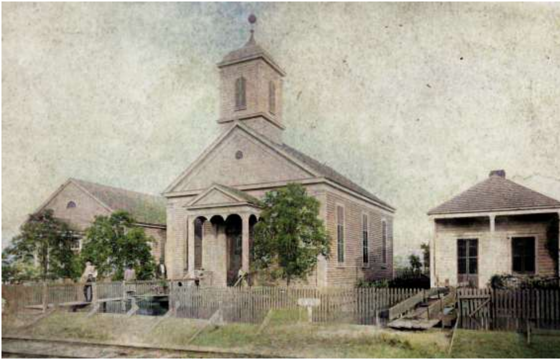
The first location of Salem Lutheran Church was on Fourth Street near Amelia in Gretna. In this photo, perhaps taken during the 1891 crevasse that flooded Gretna, the parsonage is at right of the church and the school is at the left. The congregation was founded in 1871 and this church was built the following year. (From the Historic New Orleans Collection)
